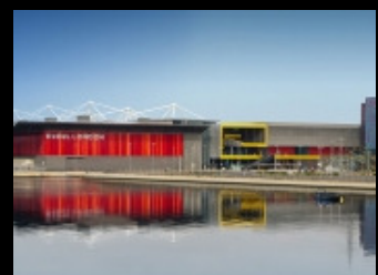
The facade from across the water.
